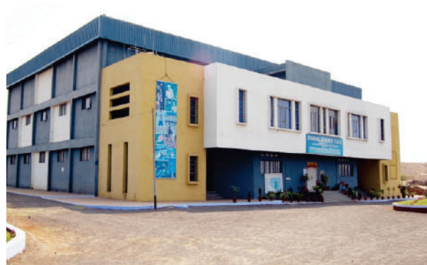
The Indoor Stadium at Rajarambapu Institute of Technology, designed to facilitate a variety of indoor sports and recreational activities, providing a vibrant space for student engagement and physical development.
