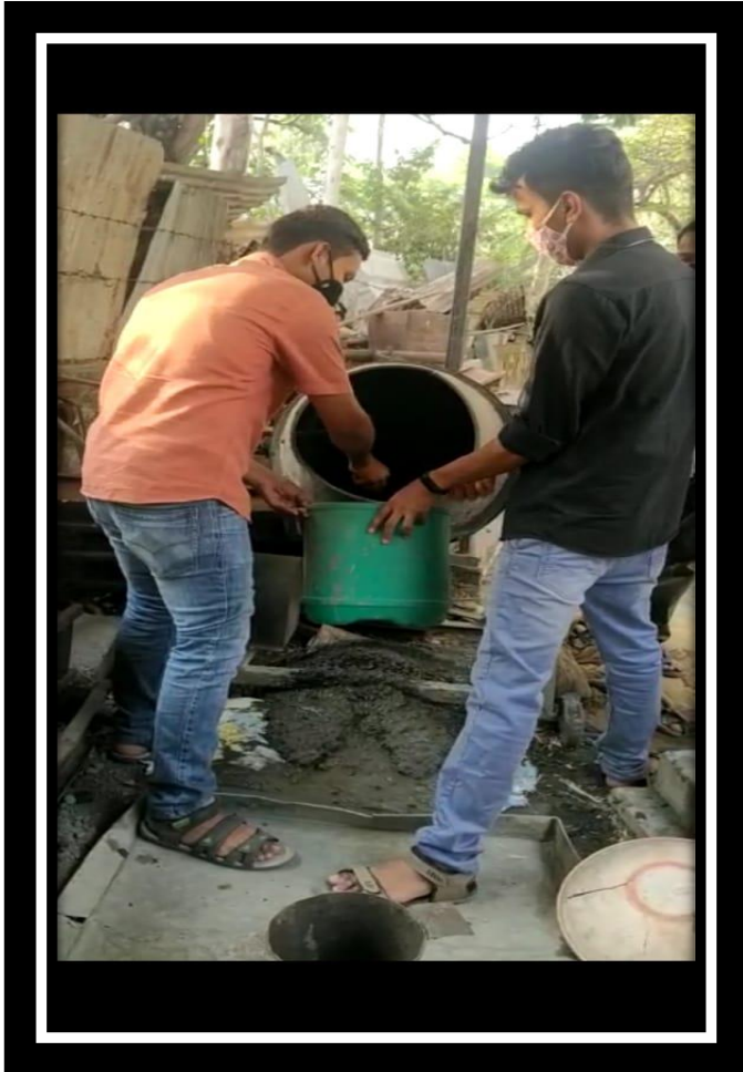
Preparation of concrete
